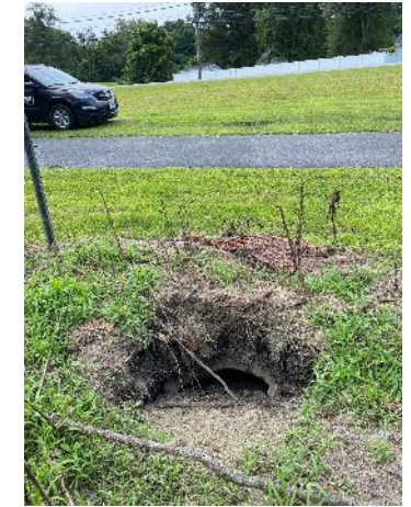
Pipe under Dorsey Rd. at Hawkins Dr.
