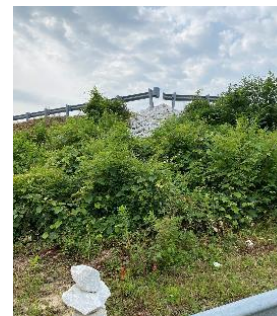
Runway 10 Glide Slope Shelter
